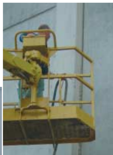
Fig. 3 Grouting on the side.
